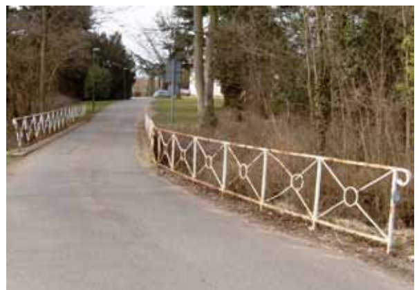
Metal balustrade to park stream at Papworth Hall
