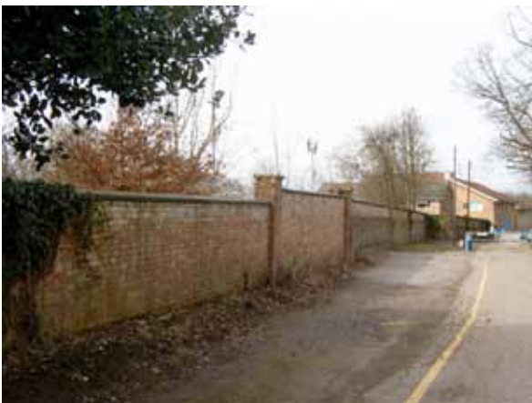
Brick wall to former vegetable garden at Papworth Hall
