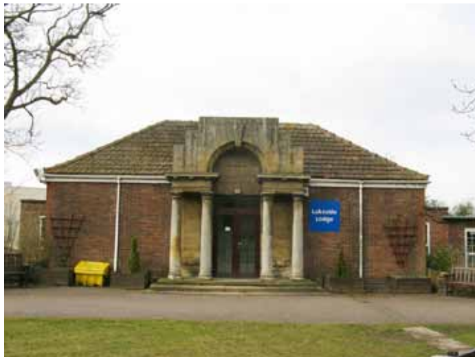
The Simms Woodhead Building (Lakeside Lodge)
