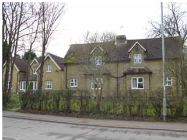
Model workers cottages on the west side of Ermine Street south
