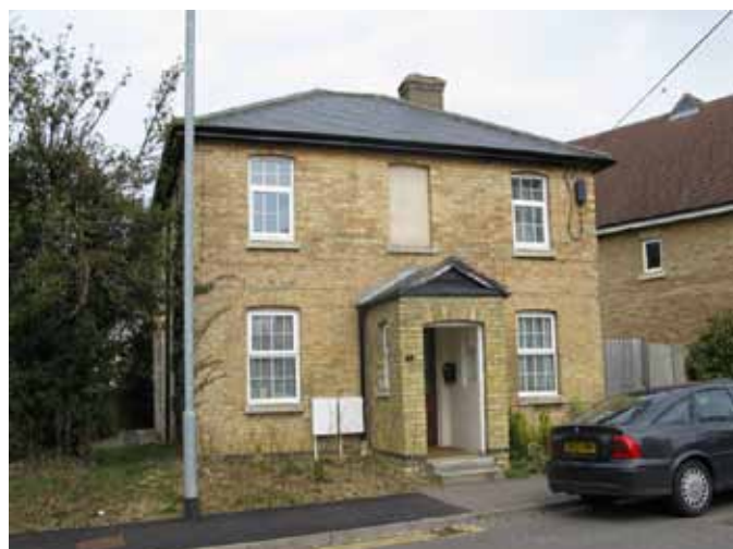
Service entrance lodge, set back from the east side of Ermine Street near to the Church Lane junction
